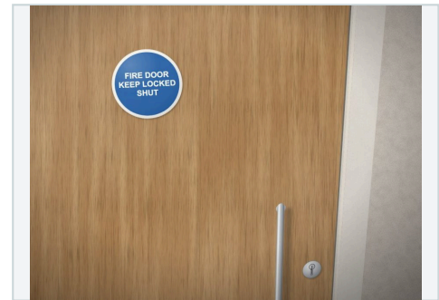
Photo 6 — The sign fitted to one face of the riser cupboard doors
